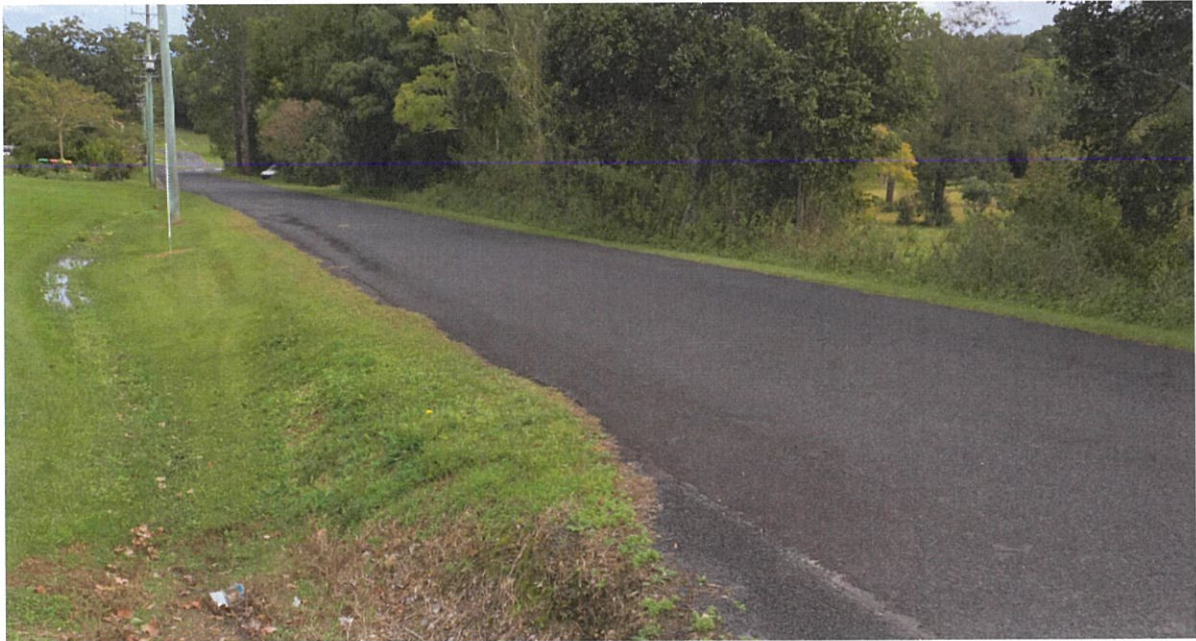
Figure 3: Rileys Hill Road looking south-west from Hills Road
