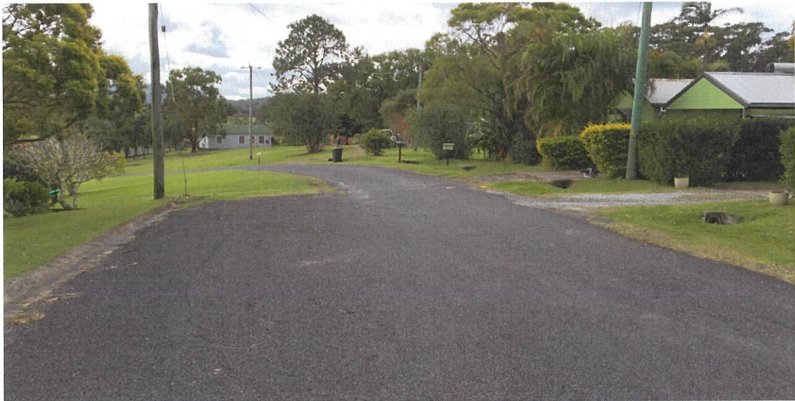
Figure 1: Hills Road looking north, showing both road standards
