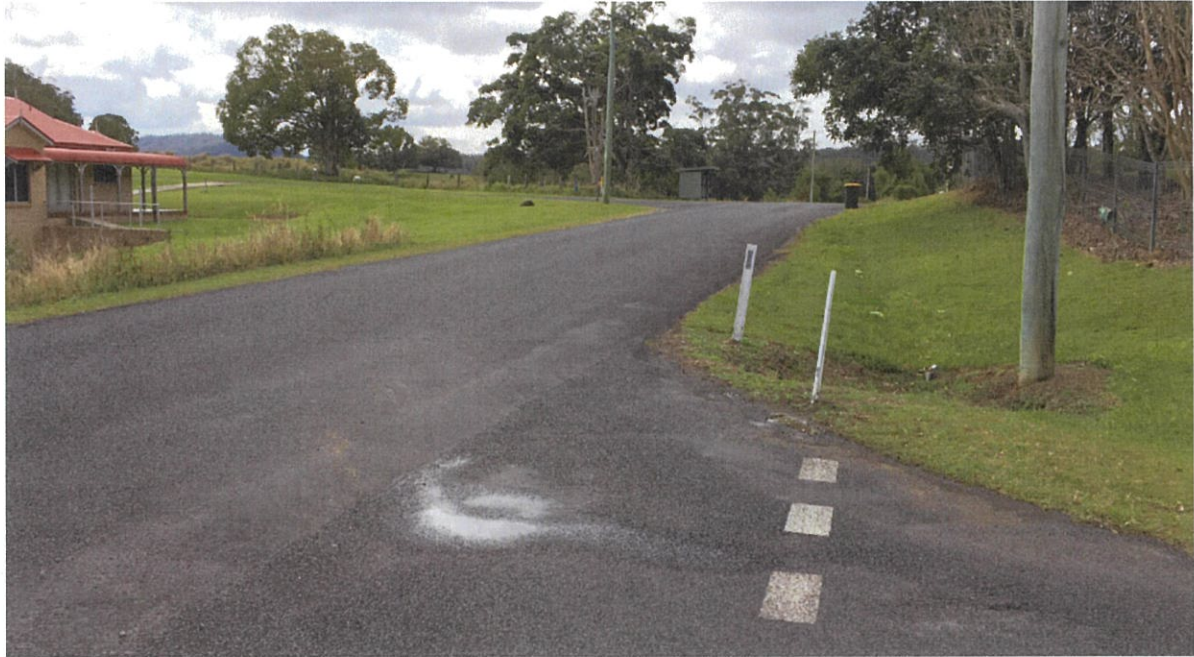
Figure 4: Rileys Hill Road looking north-east from Hills Road
