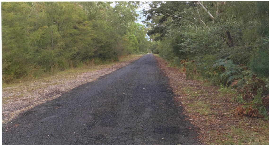
Figure 2: Hills Road south of the site entrance
